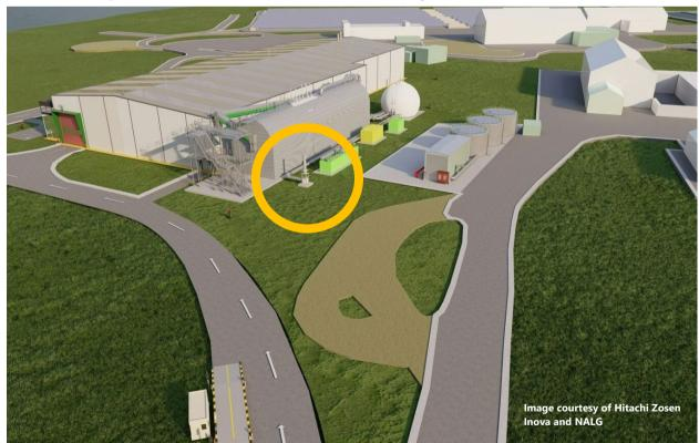
Interaction between moving vehicles and staff on site is a key safety consideration. Preventative measures such as walkways, guards, bollards, low speed limits, speed humps will be included in the facility design. A vehicle operational plan will also be developed to inform how many vehicles are allowed to be on site at once.
