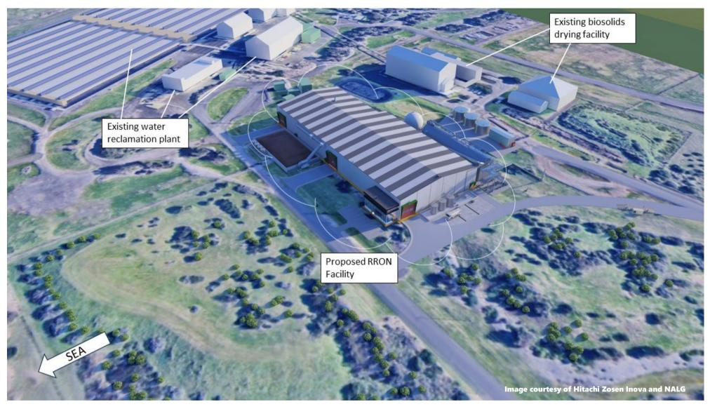
The height of the building is designed to provide enough clearance for operations, including trucks to safely drop off organic waste within the building.
