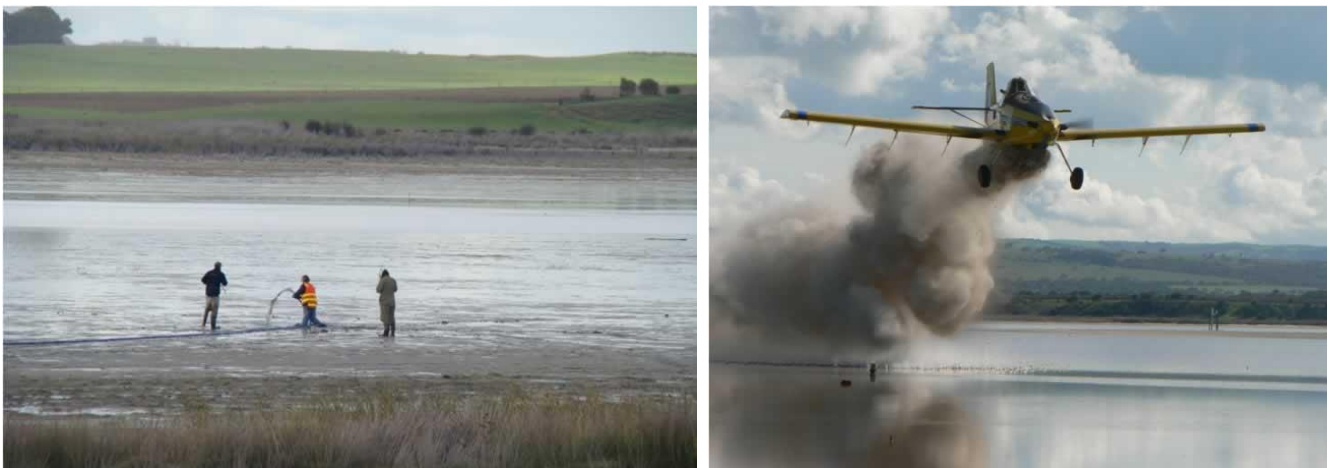
Figure 5-1 Application of slurry to Lower Murray Lakes (left) and aerial application of lime to Currency Creek (right) (EPHC & NRMCC, 2011).
