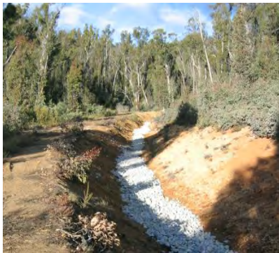
Figure 5-2 Example of open limestone drain - images from Taylor et al., 2005 (left) and Cravotta 2010 (right)
